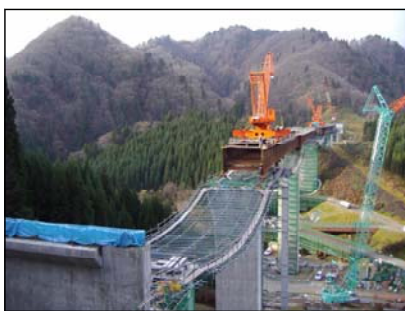
(桁架設状況・H19.11)
