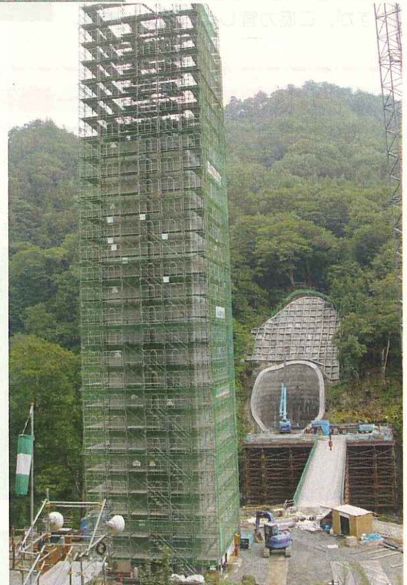
(P2橋脚施工状況)
