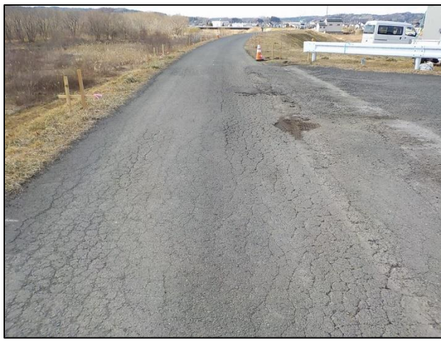
堤防天端舗装(浅水川付近)【打換え】前
