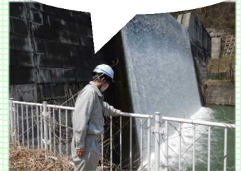
▲入間砂防堰堤
