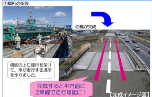
①橋桁の架設
