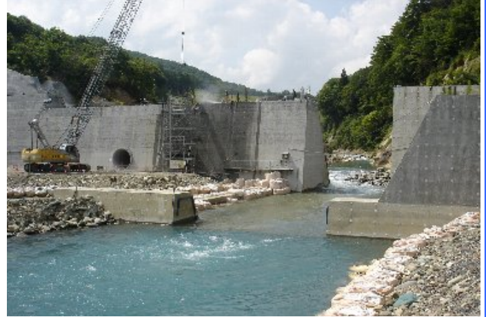
◎市野々原2号砂防堰堤
